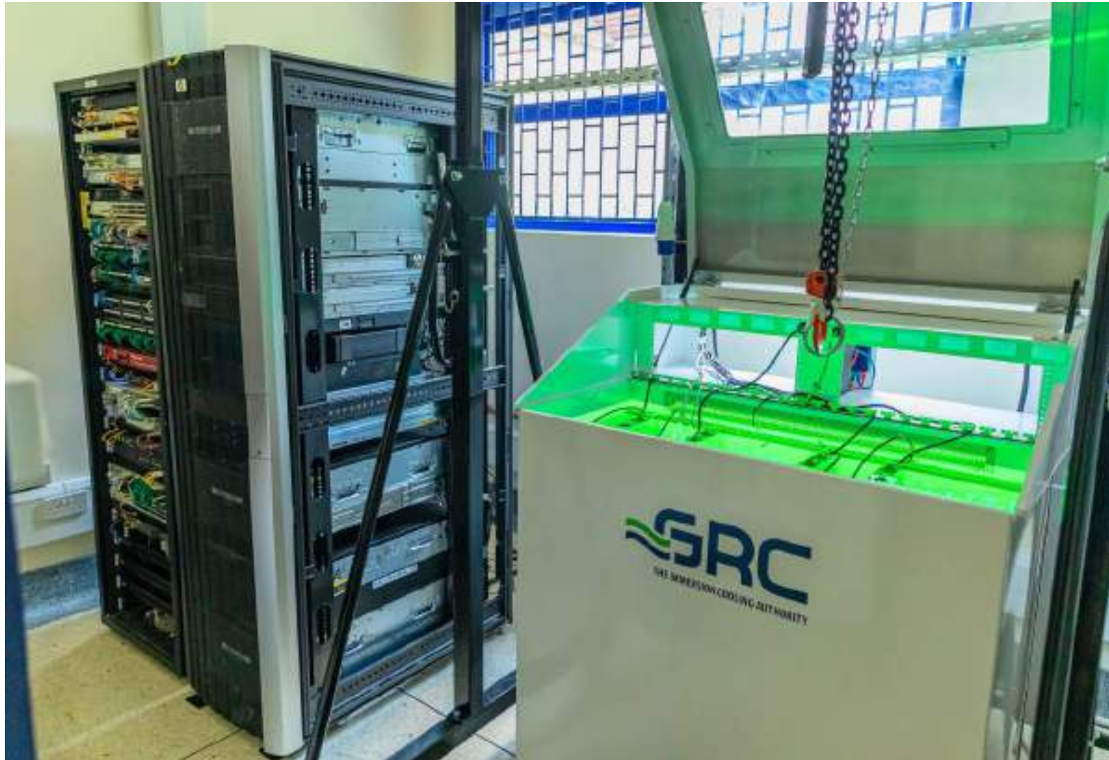
Immersion cooler for servers at RHSP premises.
